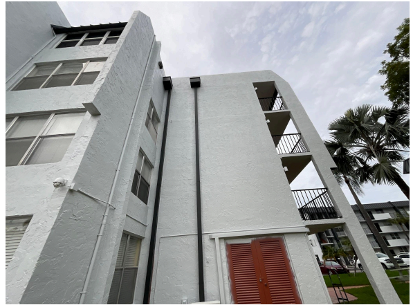
Building exterior surfaces, rain gutters and doors
