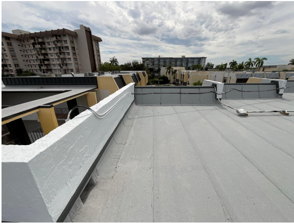
Rolled modified bitumen flat roof
