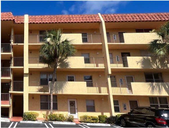
Building exterior stucco and railing
