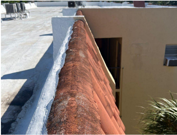
Tile mansard roof
